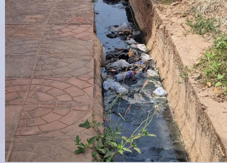
Fig 3. Clogged Drainage System
