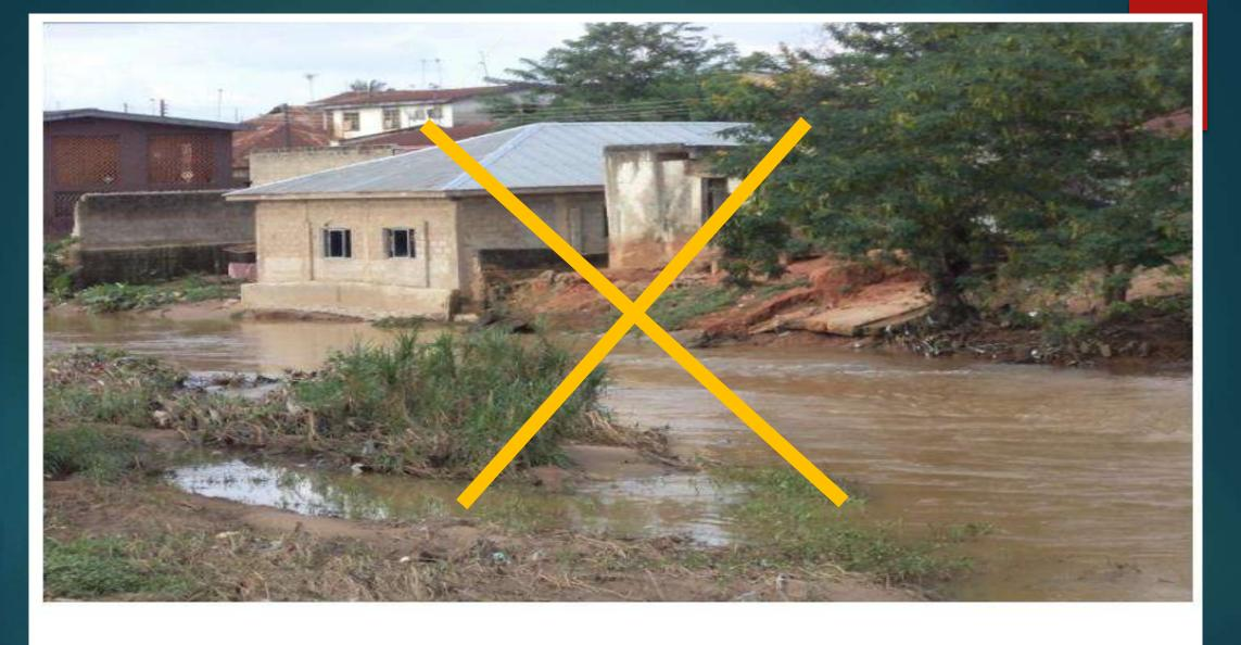
Construction on River Flood Plain – Odo Ona Area Building constructed right within the river channel
